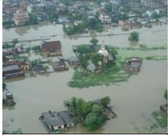
Aerial view of floods in the affected area
