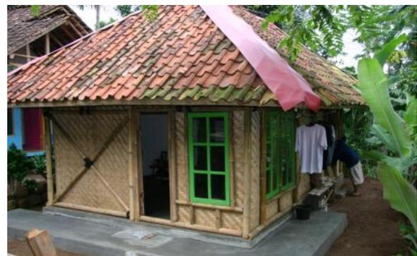
In West Java, construction with bamboo is still widely practised, both for framing of livestock pens, temporary buildings and restaurants. The use of woven bamboo sheeting remains common for both internal and external walls in rural or poorer housing. (Photo by: IFRC)
