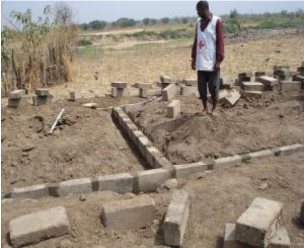
Foundation casting stage
