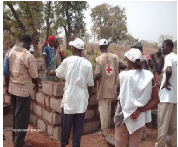
Brick laying stage
