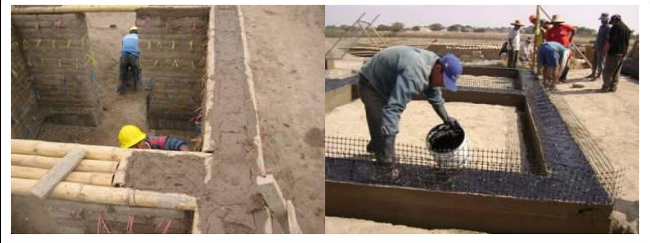
2. After levelling the ground and setting stone foundations, adobe brick walls and columns are raised. The materials and the design have the additional advantage of a natural heat insulation system. During mornings, the walls gather heat from the sun, keeping the house interior cool, and liberate heat during cold nights. The whole building is reinforced with cane structures. Plastic bonds are placed with every each three brick layers to tighten the geogrid, which will envelop the walls.
