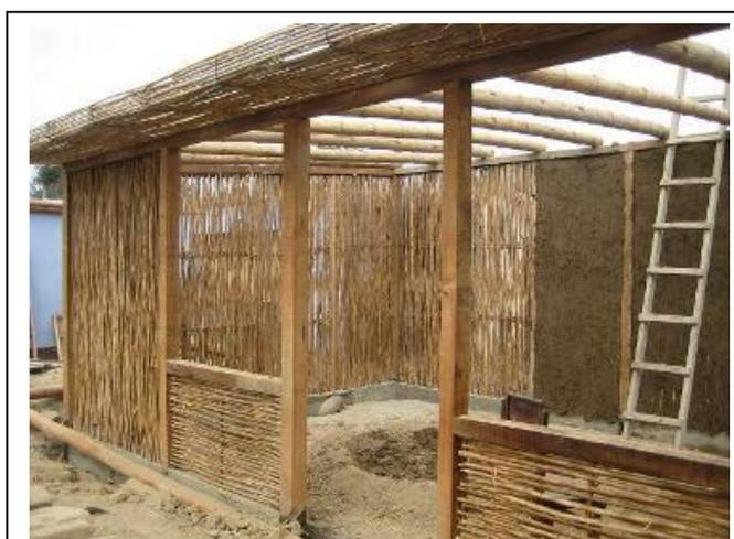
The first 15 of one 120 permanent seismic-resistant *quincha* houses are being built in Northern Bernal. The improved traditional *quincha* consists of reinforced reed structures plastered with mud. The construction techniques employed by the International Federation have the additional advantage of efficient thermo-insulation. Source: International Federation
