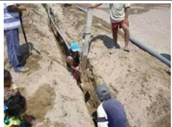
Water pipes being installed by the community in Villacurí. Members of the Movement, such as SRC and GRC, have implemented water and sanitation programmes. Source: German Red Cross.
