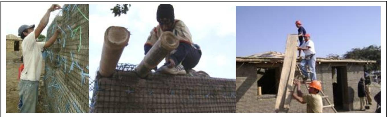
3. Combined with cane flexibility, the geogrid is the base of the self-supporting structure and seismic resistance. The picture shows this final tightening of the geogrid, prior to the mounting of the ceiling. This will be covered with a cement layer to ensure durability.
