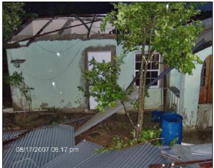
Dean has left many houses severely damaged. Source: Saint Lucia Red Cross
