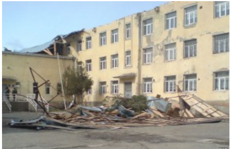
Heavy wind removed the roof from the residential building, Gori. Photo: Georgia Red Cross
