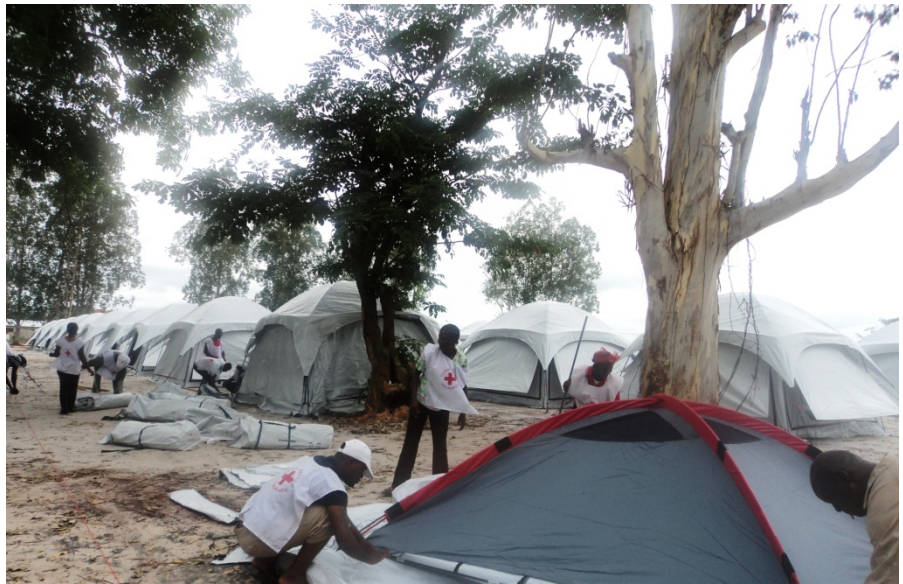
Congolese Red Cross volunteers erected tents to help accommodate the vulnerable people that were left homeless after the explosion and destruction of their homes. Photo/Josuane TENE - IFRC
