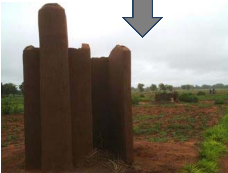
Example of toilet improvement in Ukoto B before (above) and after (below) the DREF Operation;
