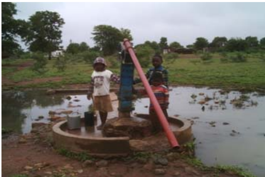
Barefoot children at a disfunctional borehole in Ward 20 potentially using the unsafe water in the open pools. Photo ZRCS
