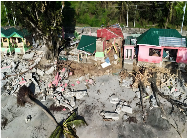
1 Destructive winds brought by Typhoon Uwan (Fung-wong) tore off roofs and uprooted trees along the coastal area of Dipaculao, Aurora. (Photo: PRC)
