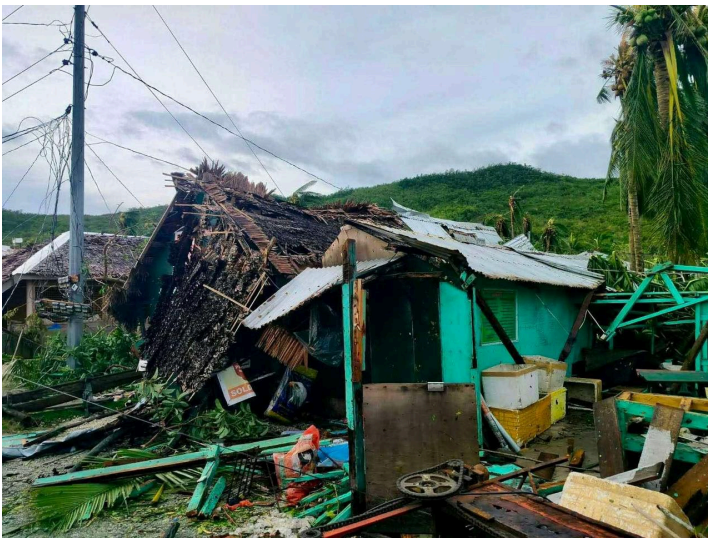
Damaged house due to Typhoon Tino in Dinagat Islands. (Photo: PRC)
