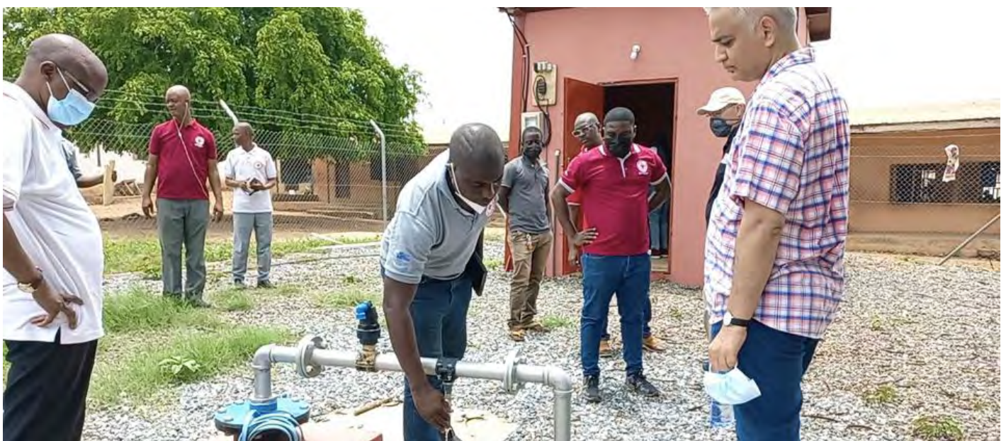
National Society volunteers constructing water supply systems across communities in Eastern and Ashanti regions in Ghana. (Photo: IFRC)
