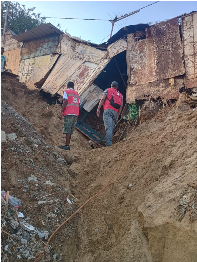
Destruction in Sao Vicente after the floods and strong winds of 10 August 2025
