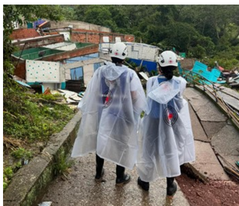
Damage assessment San Cristóbal branch. 24 June 2025. VRC
