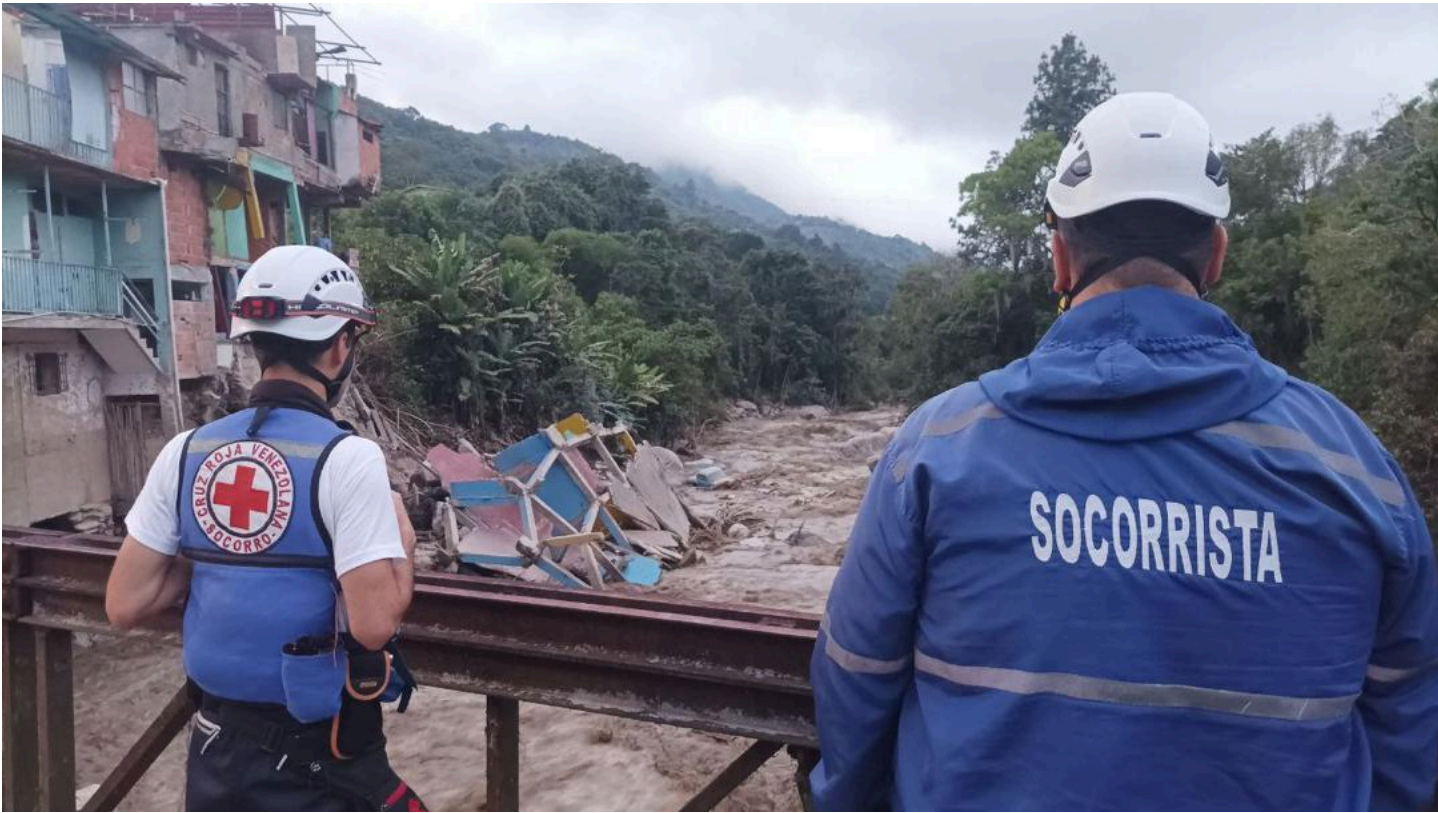
Damage in Arenal (Edo. Mérida) 26 June 2025. Source: Mérida Branch,
