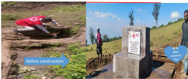
Pictures of water points development under process
