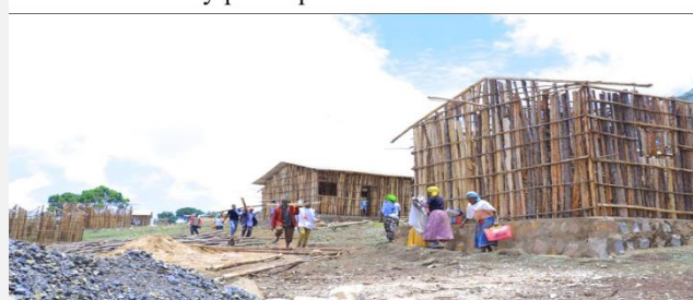
Community participation in shelter construction
