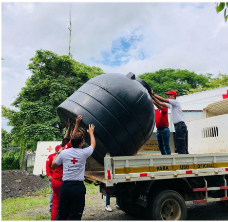
Installation of safe water storage tanks. June 2025. Source: RCSP
