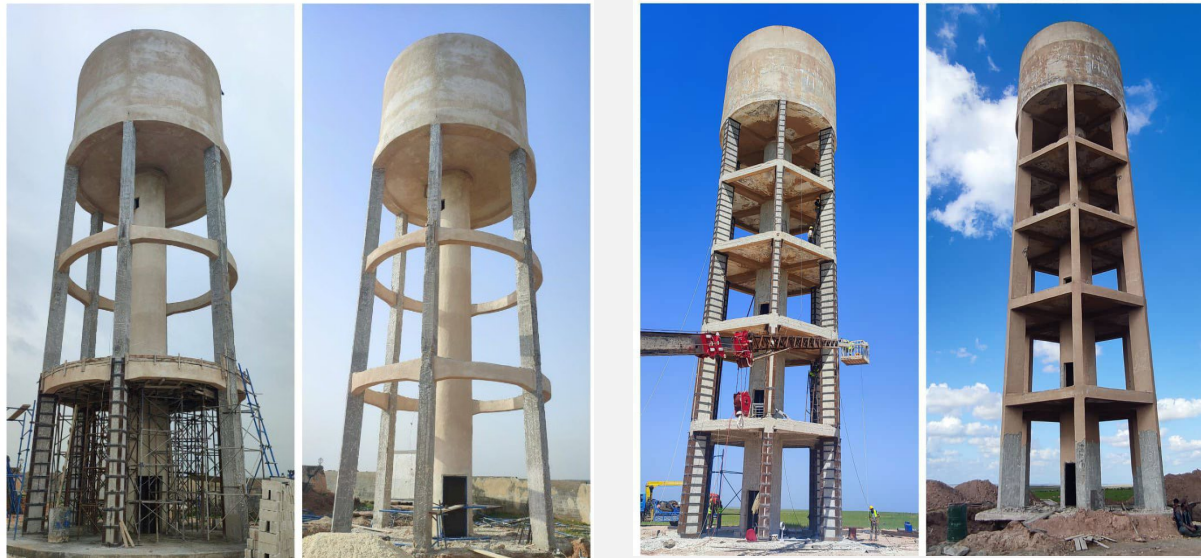
Rehabilitation of the elevated water tanks in progress
