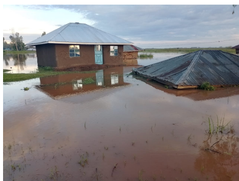
Destroyed household by the ongoing floods
