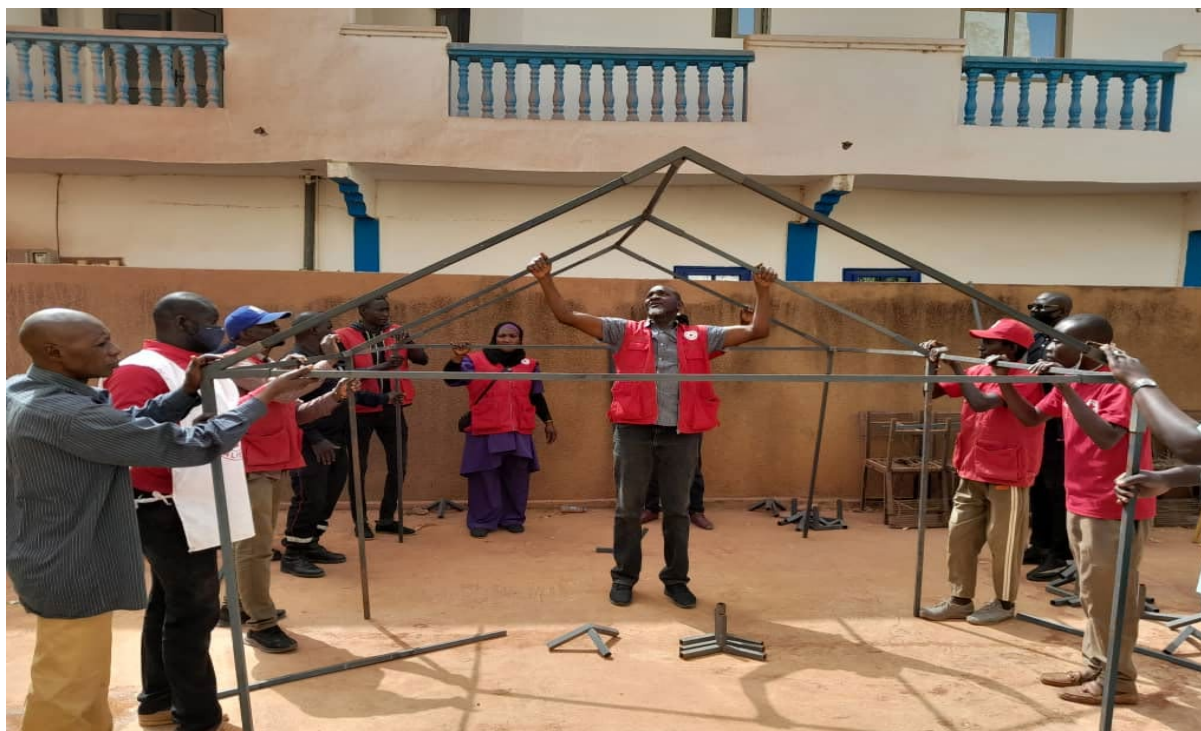
Demonstration of shelter construction in Segou (source Mali Red Cross)
