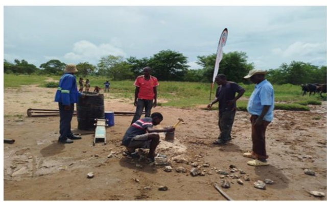
Community members assisting in borehole rehabilitation
