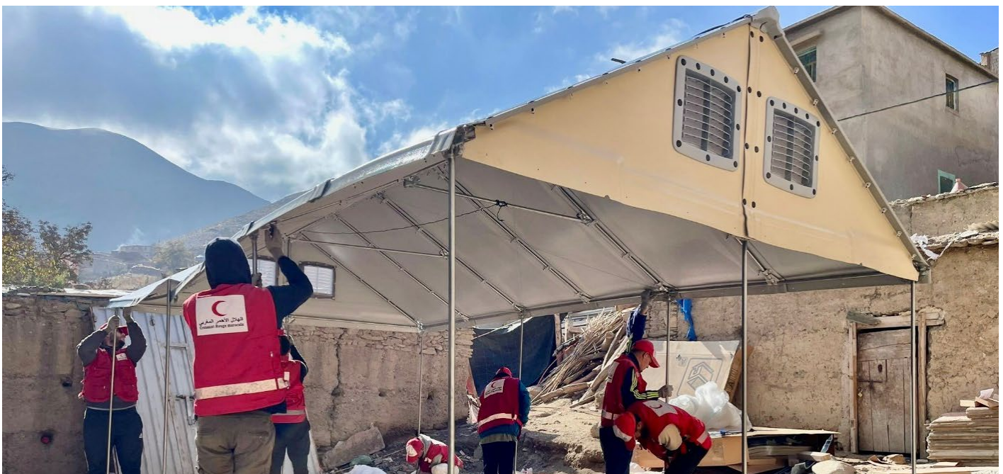
Photo 1 – Chichaoua – Shelter activity – concrete pocket anchoring, TSU installation, flooring and insulation – Nov. 2024 (Photo: MRC / IFRC)
