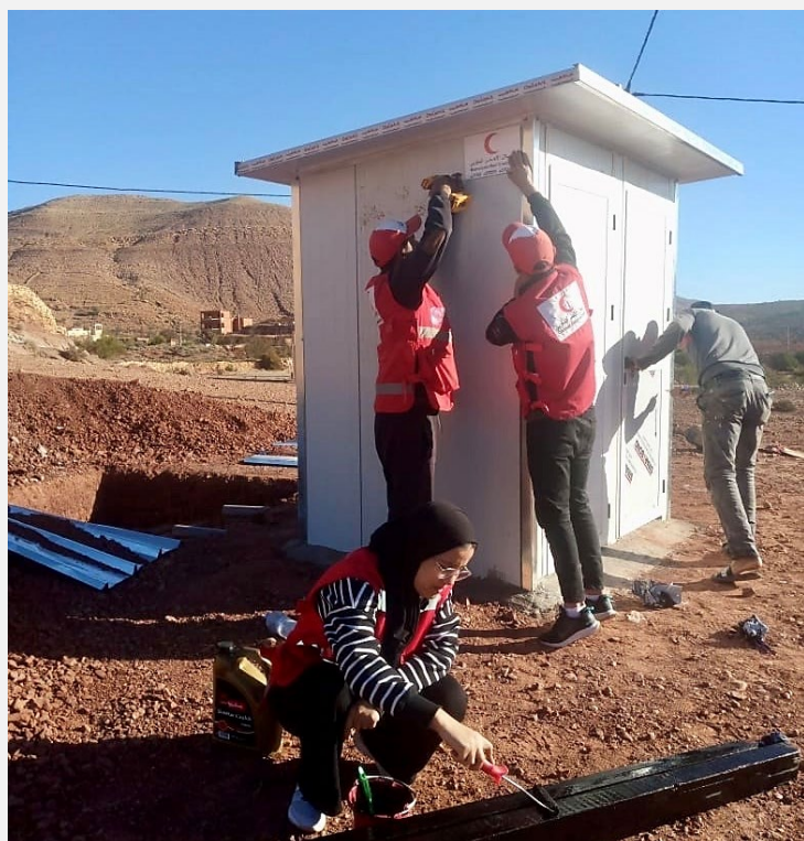
Photo 9 - Photo - Installation of toilets modules for Chichaoua schools (November 2024)
