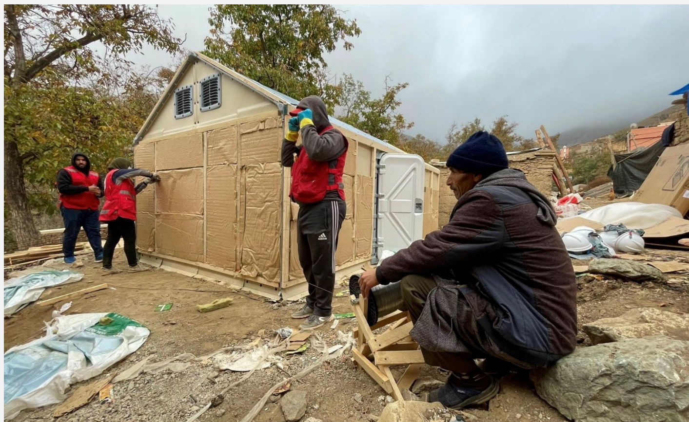
Photo 4 - TSU insulation and flooring in Chichaoua (November 2024)
