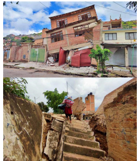
Destroyed housing and collapsed public infrastructure in Nuevo Amanecer, Cochabamba, March 2025. Source: Los Tiempos
