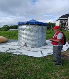
After the earthquake, upon arrival at the plant, it was observed that the 12,000-liter Oxfam tank had a slight tilt and some minor damage but remained operational. An action plan was established to carry out the repairs without interrupting operations.
