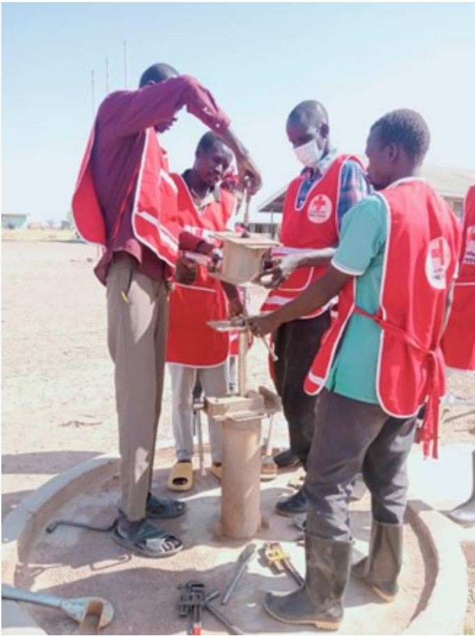
SSRC Rehabilitating Water point
