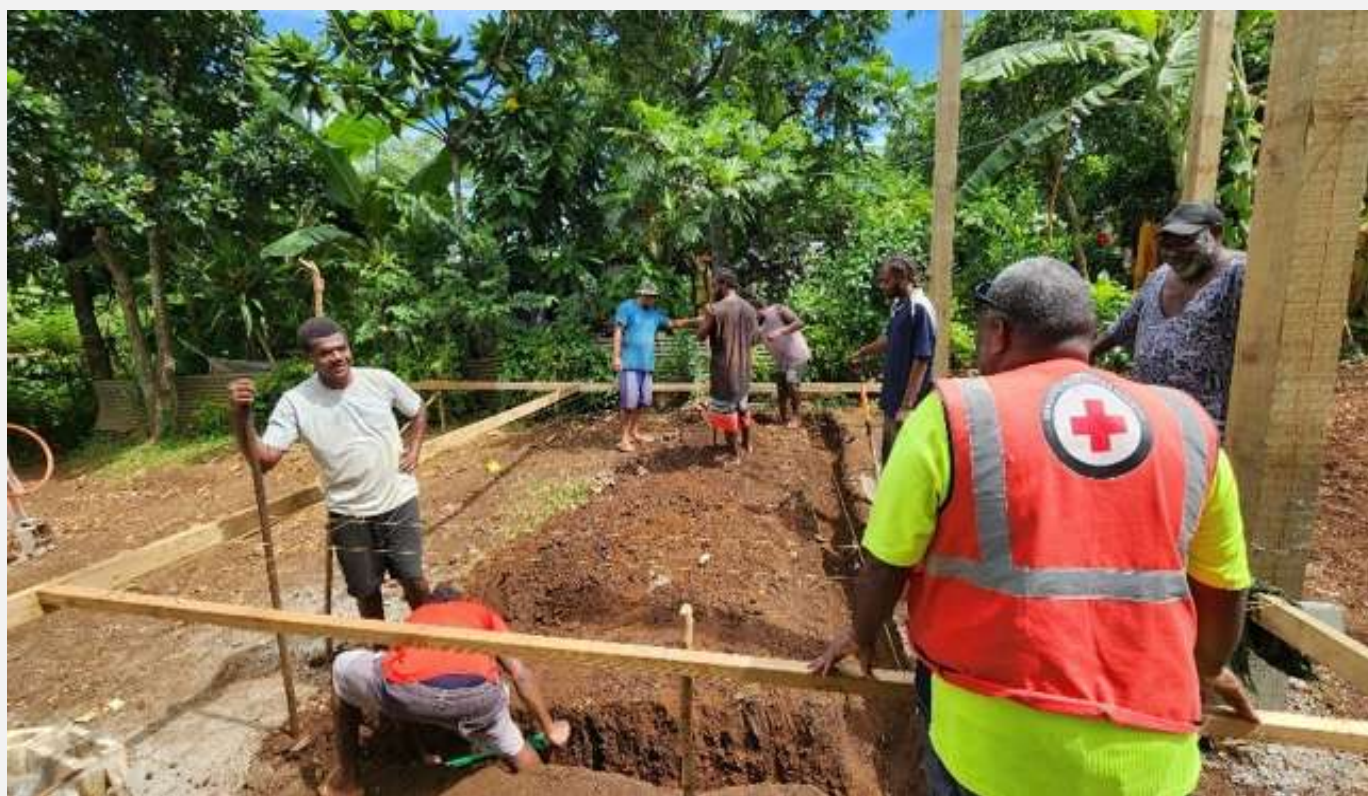
Red Cross volunteers and community members working together to construct a water catchment system in Britano Community, improving access to safe water for families (Photo: VRCS)
