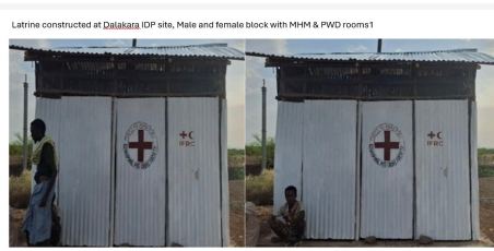
Latrines constructed at Dalakara IDP site
