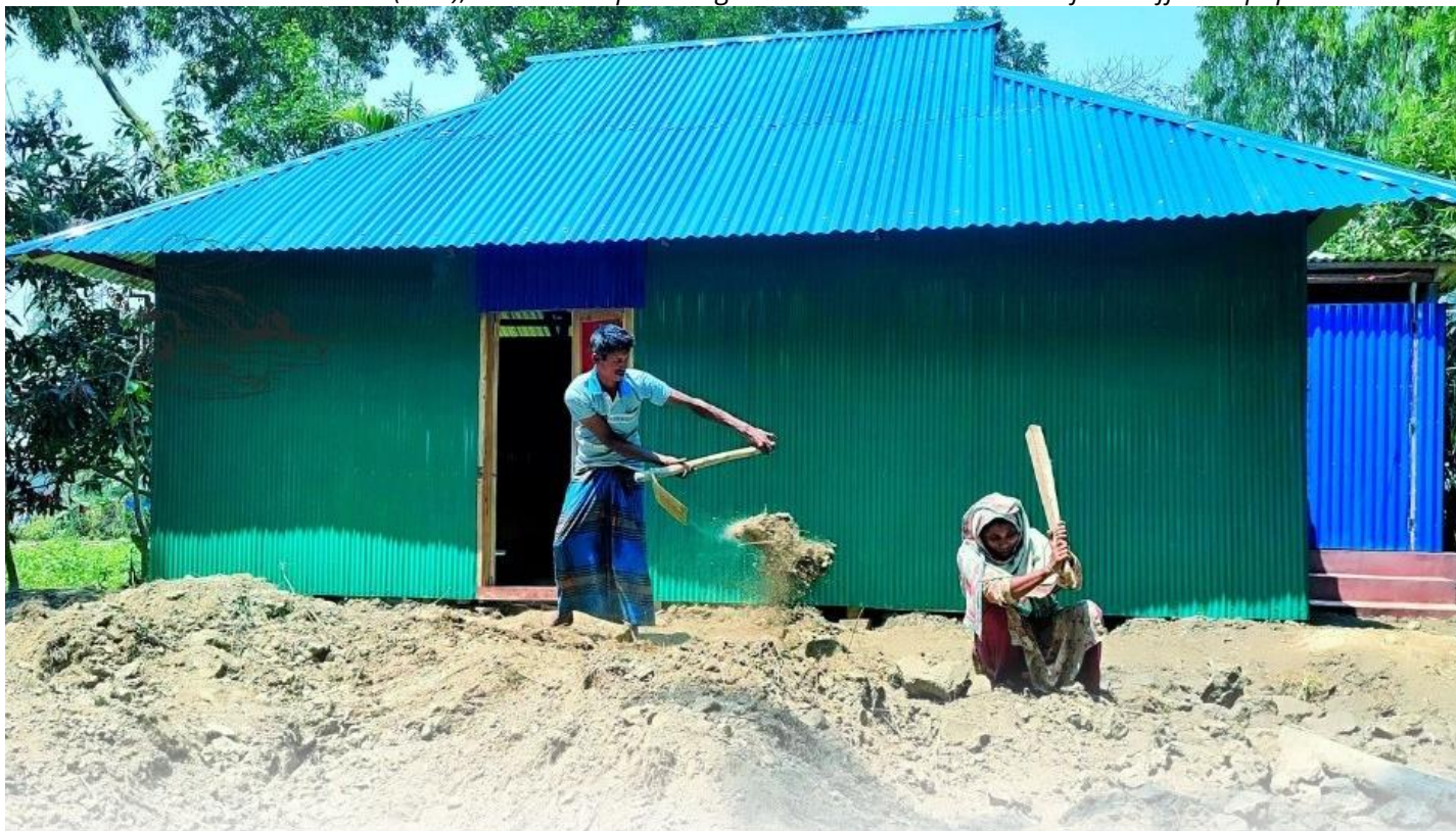
With support from BDRCS through conditional cash assistance for shelter recovery, community members work to rebuild their home in Feni district. (Photo: BDRCS)
