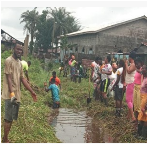
Community drainage cleaning
