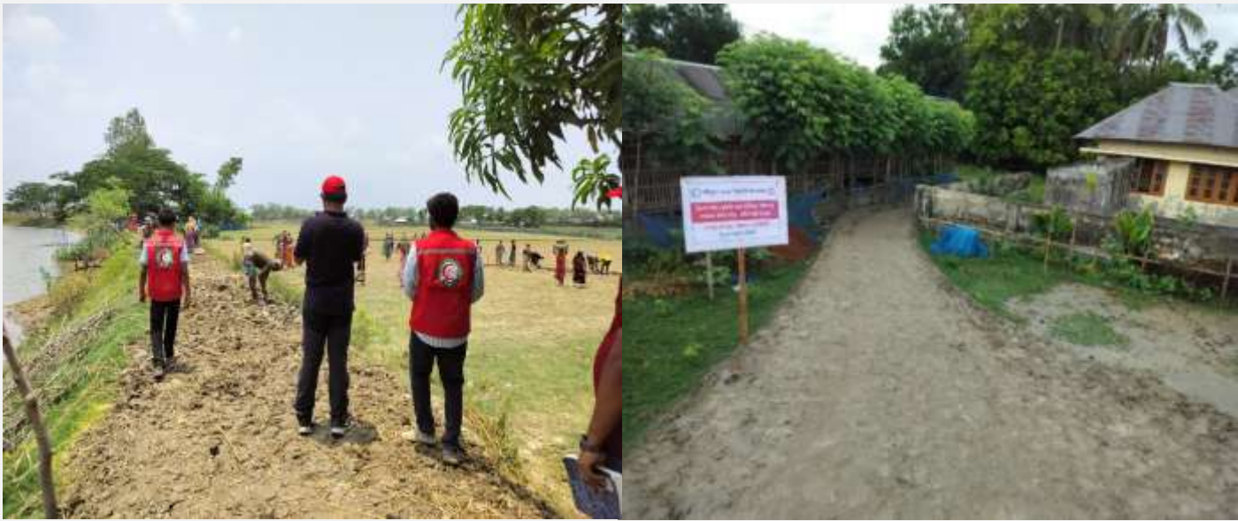
Before and after: Improvements of one of the community roads made through the Cash for Work schemes in Khulna District (Photo: BDRCS)
