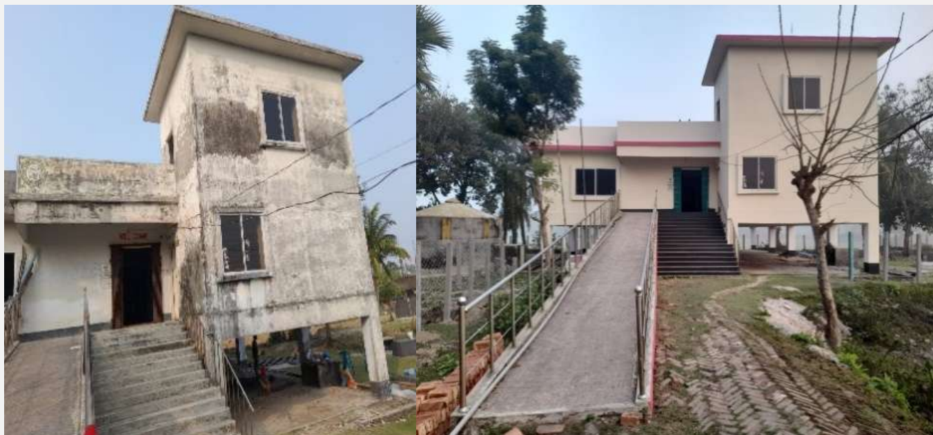
Harinagar MCH Centre in Satkhira: A transformation from deterioration to renewed care through comprehensive renovation (Photo: BDRCS)
