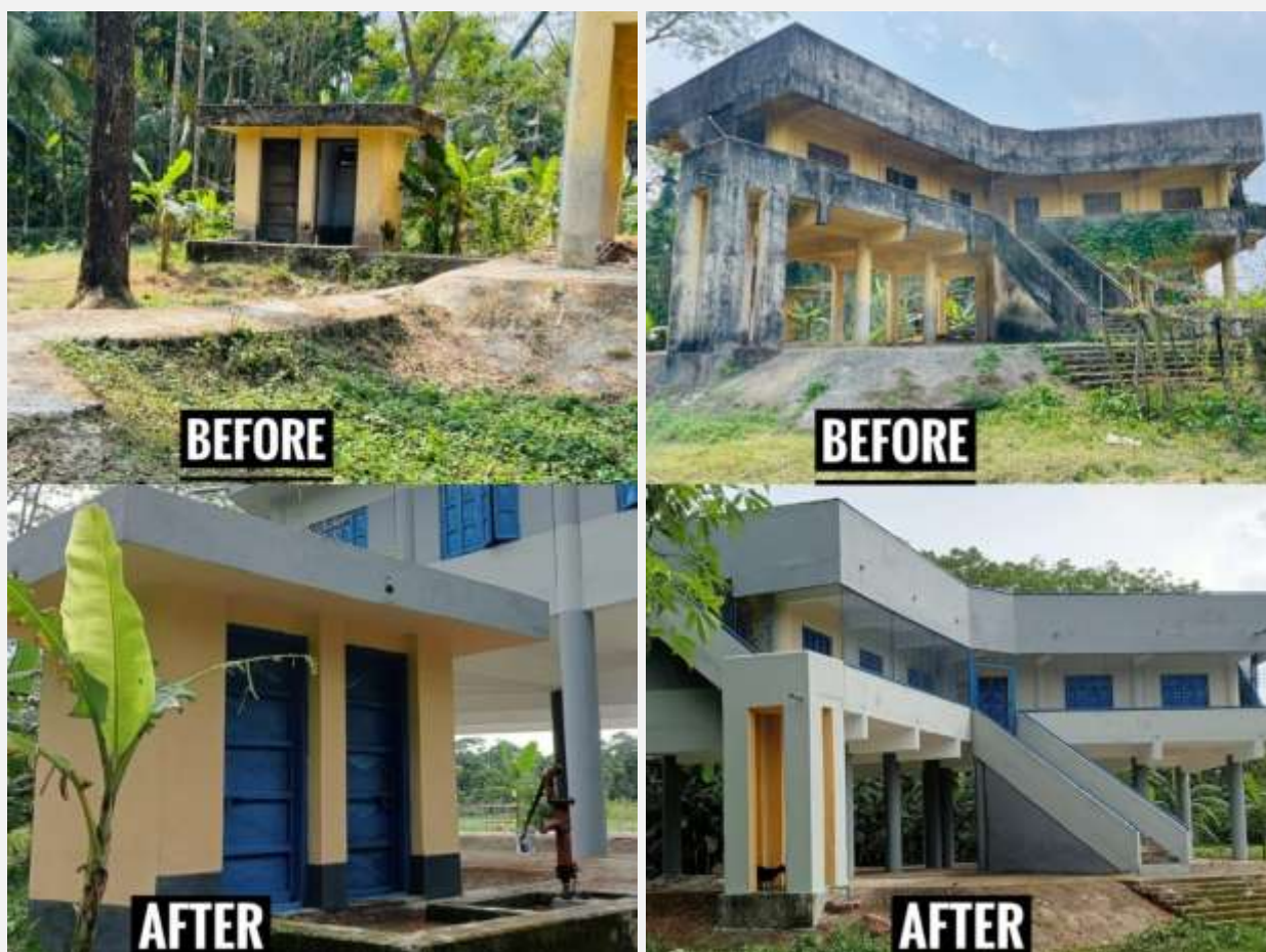
Renovated Cyclone Shelter in Indurkani Upazila, Pirojpur District – A resilient safe haven restored by BDRCS (Photo: BDRCS)
