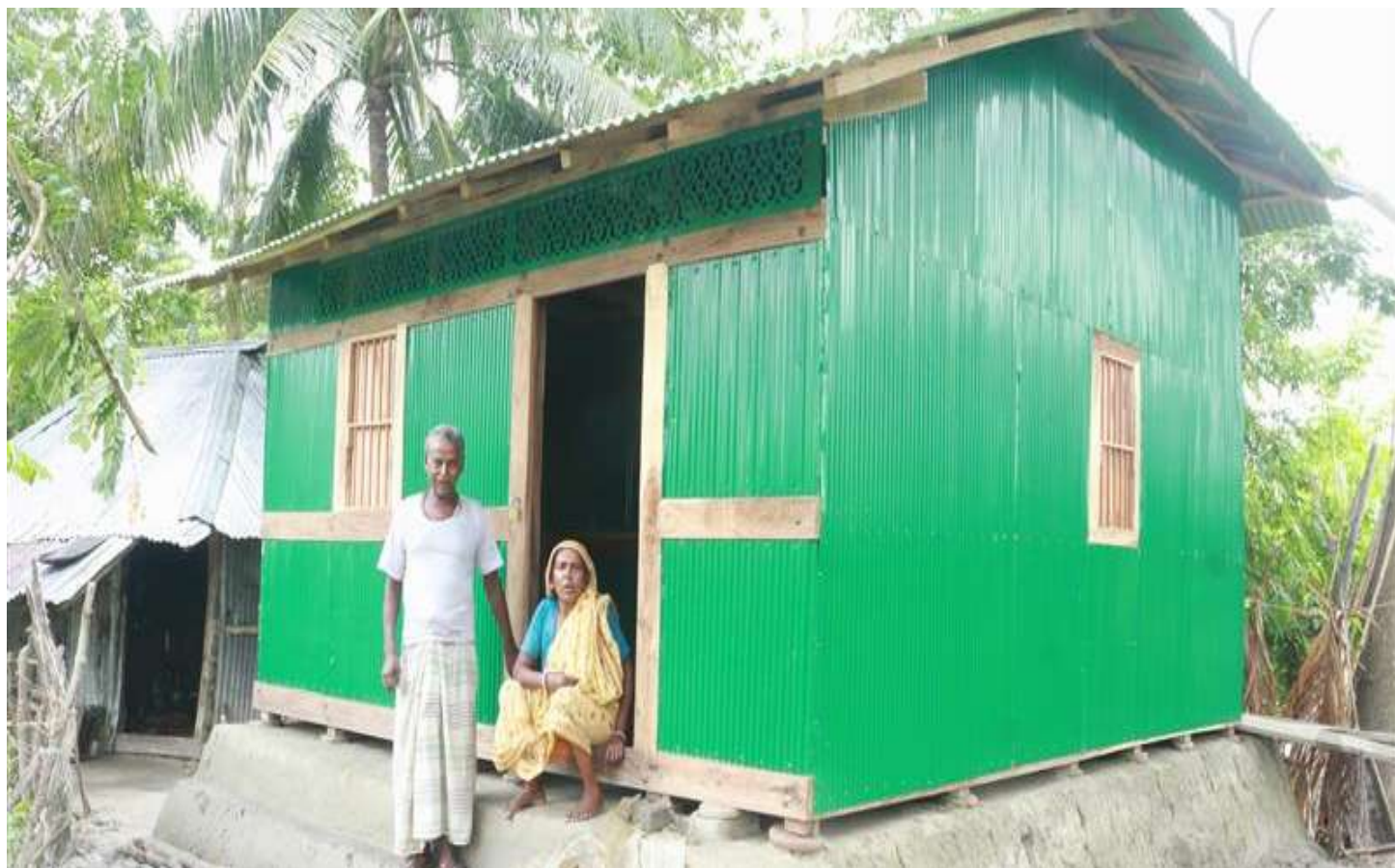
A new beginning after the storm; this family proudly stands in front of their new home, built with hope and support from the Cyclone Remal operation. (Photo: IFRC)
