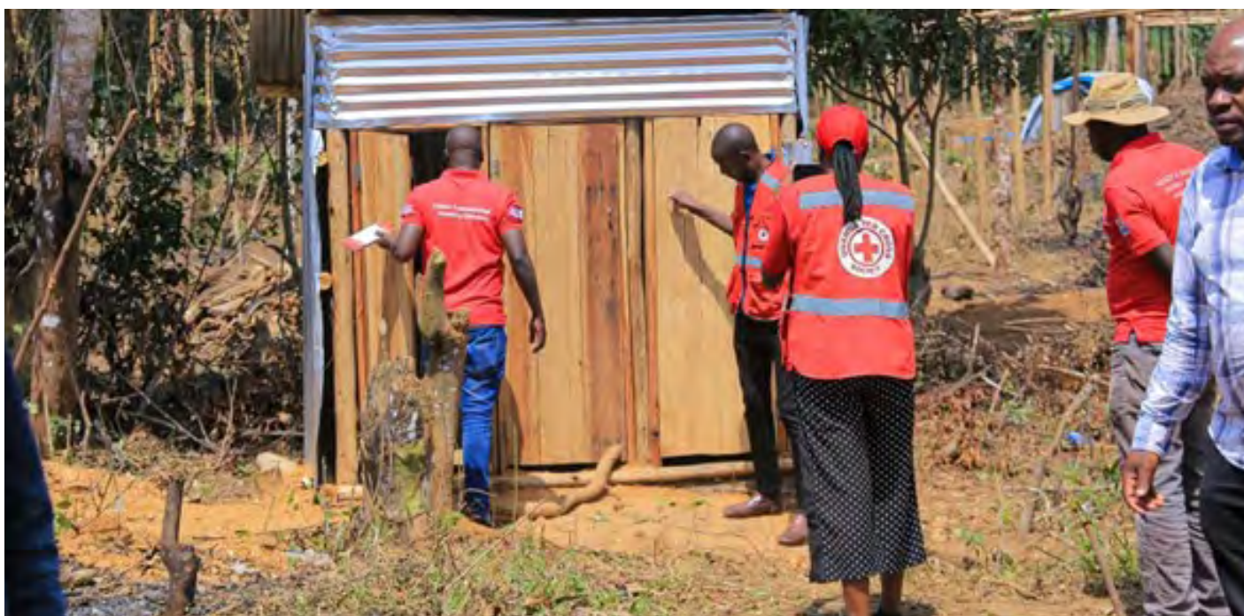
Uganda Red Cross Society team assessing the condition of the existing latrine at a camp for internally displaced persons (Photo: Uganda Red Cross Society)
