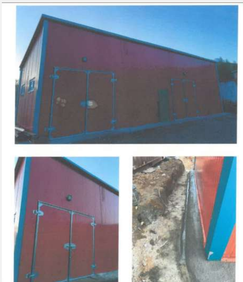
Warehouse after completion, November June 2025 (Photo: MRCS)
