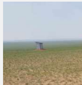
Beneficiaries installed their pit latrines in their winter shelter area (Photo: MRCS)
