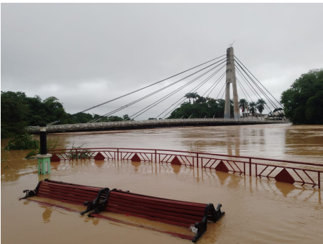
Impact of the floods on the Wilson Pinheiro Binational Bridge. Rio Acre, Pando, Bolivia. March 2024. Source: Bolivian Red Cross
