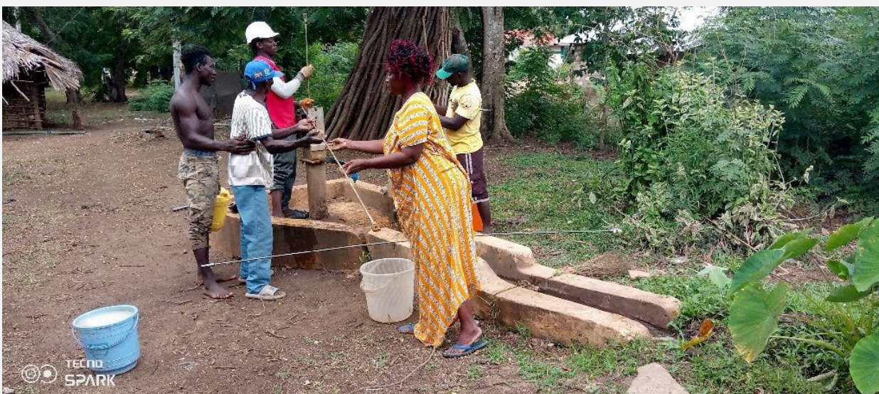
Hand pump under repair in Tana River (KRCS photo)
