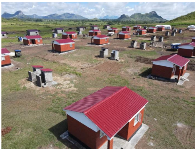
Newly Constructed TC Freddy Houses Chiradzuru District
