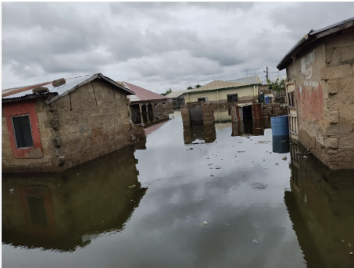
Floods September 2023, Buipe Town in Savannah region (Ghana)- by GRCS
