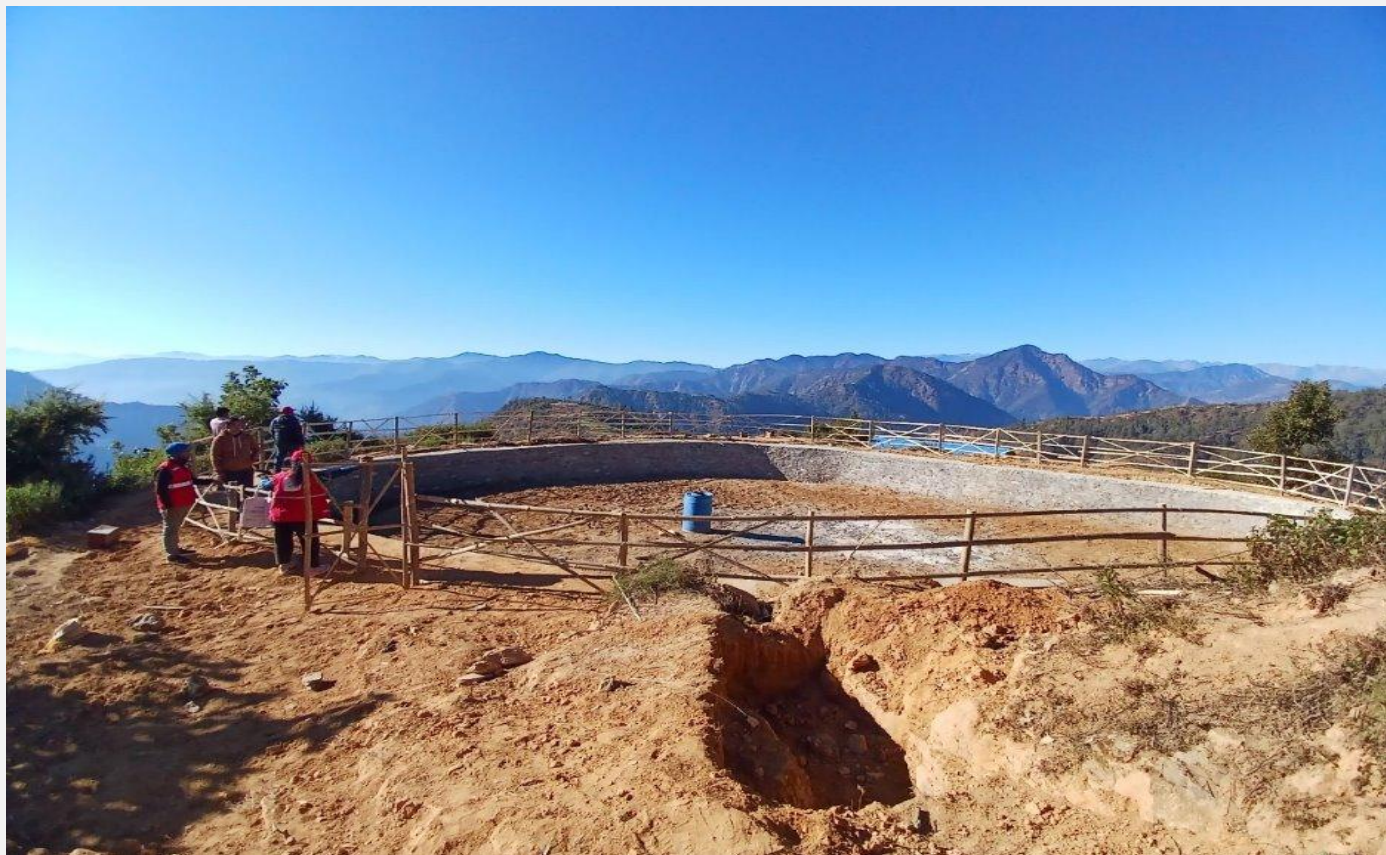
A completed mitigation scheme at the top of the hills of Rukum West district, which will help to restore water recharge. The water will be collected during the monsoon season and will help in restoring the groundwater level. (Photo: Shailesh Shrestha, NRCS)
