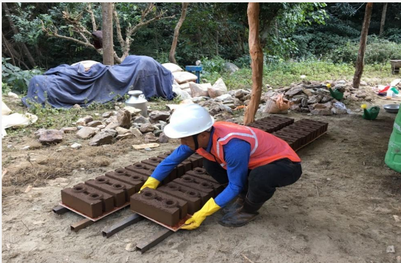
The compressed stabilized earth blocks are installed in two locations of Jajarkot which will start selling blocks for construction once the permanent shelter construction is started. (Photo: Manish Timsina, NRCS)
