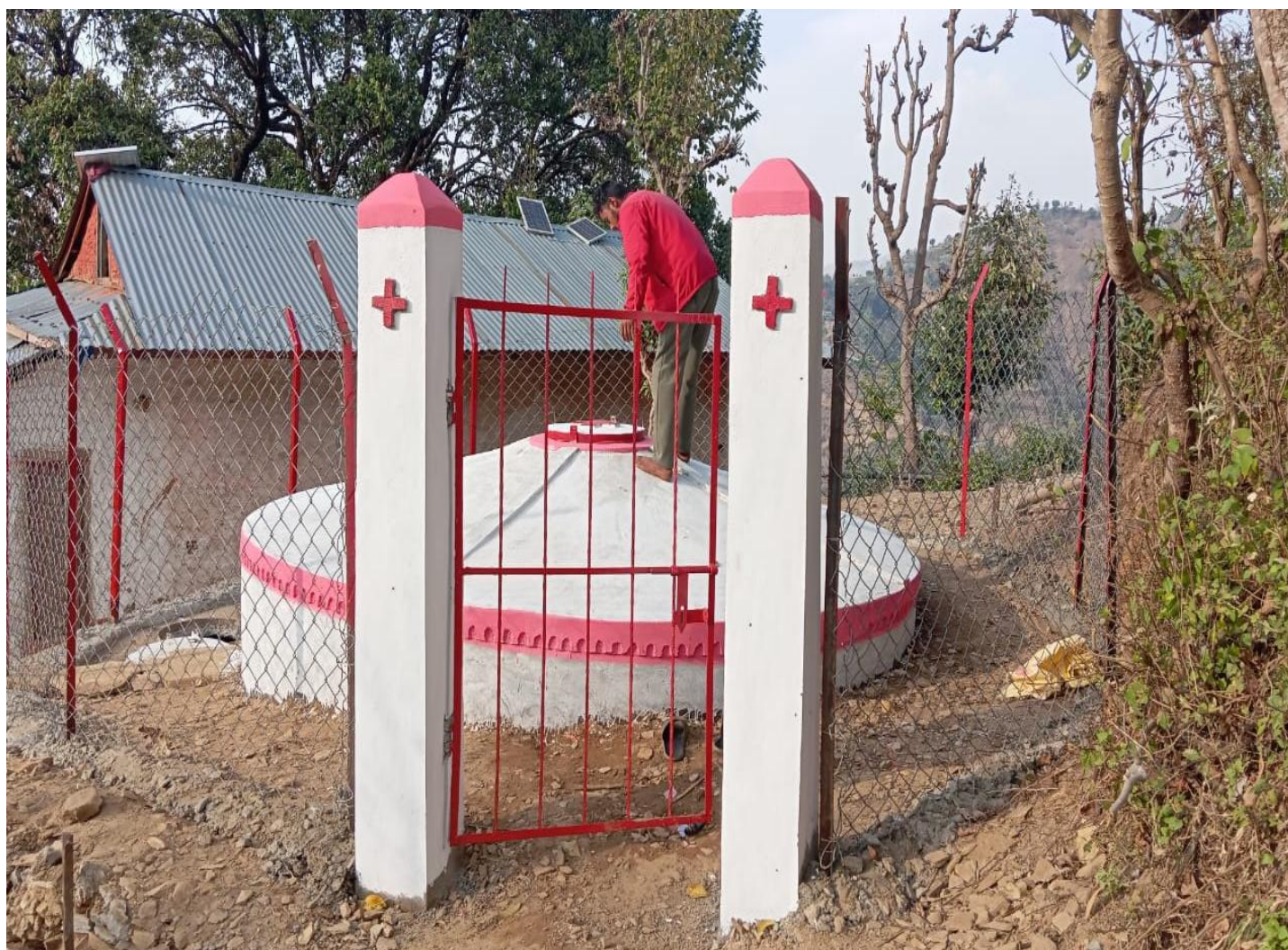
A completed water scheme in Salyan district with the support of the IFRC Network as part of the Karnali EQ Operation. (Photo: NRCS)
