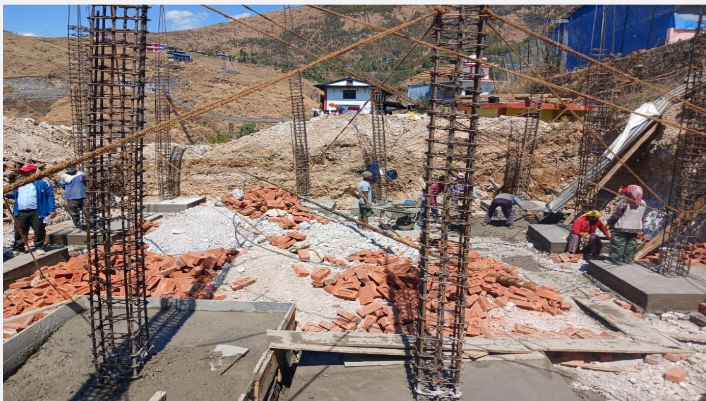
Ongoing office building in Rukum West in March 2025. (Photos: NRCS)
