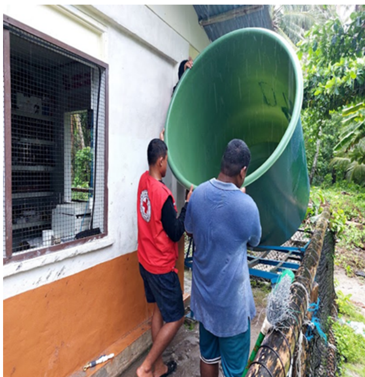
Installation of Water tank for rainwater harvesting. (Photo: MRCS)
