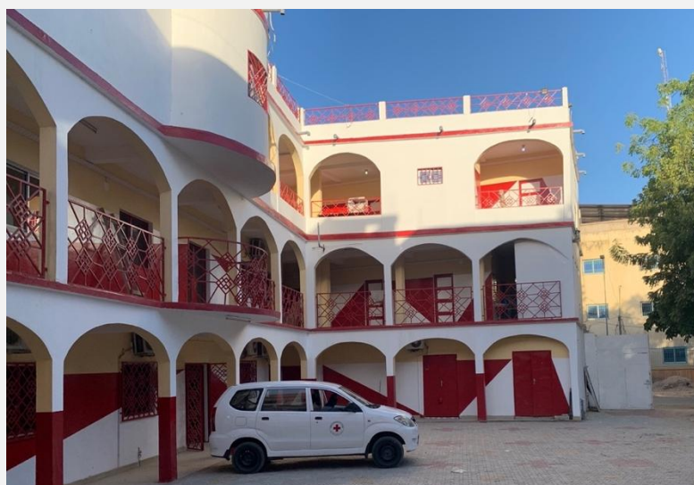
Partial image of the renovated national headquarters
