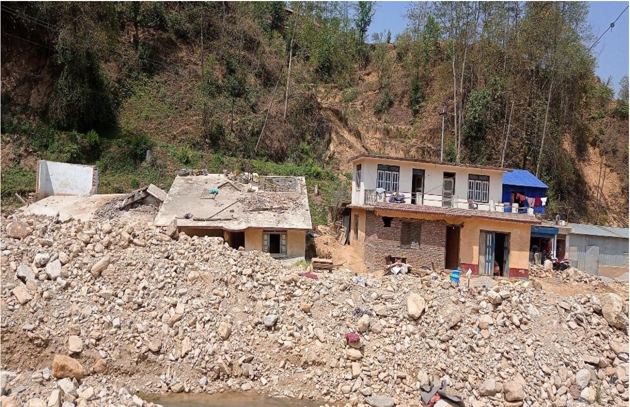
Flood impact in Panauti municipality, Kavrepalanchowk
