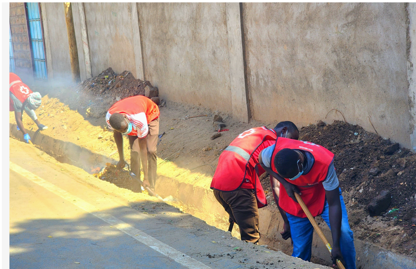
Kenya Red Cross Volunteers Supporting Drainage Clearing Ahead of the El Nino
