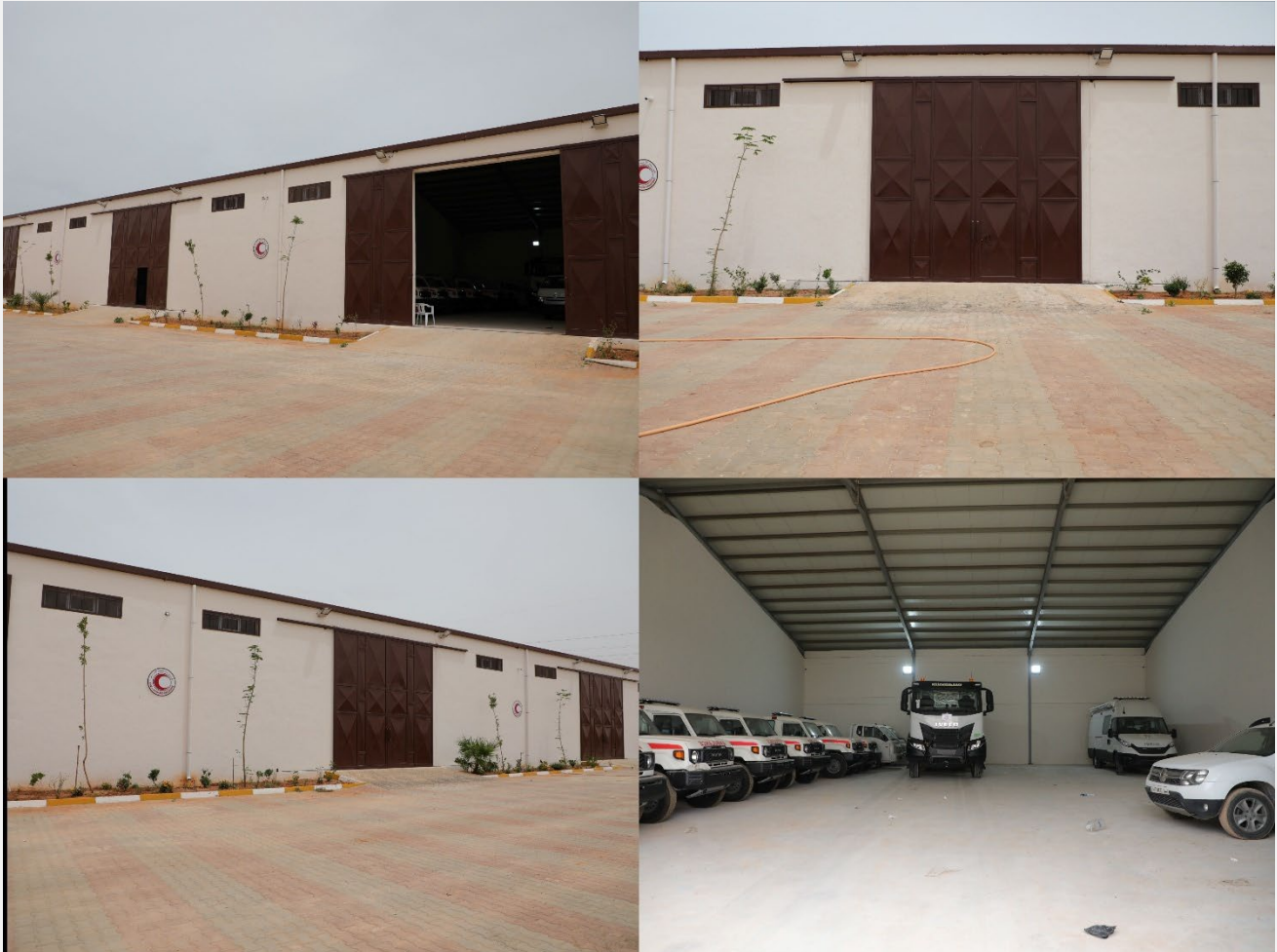
LRCS main warehouse in Benghazi (Bouatni area) post rehabilitation, with improved structural integrity, safety systems, and readiness for humanitarian logistics and emergency response.
