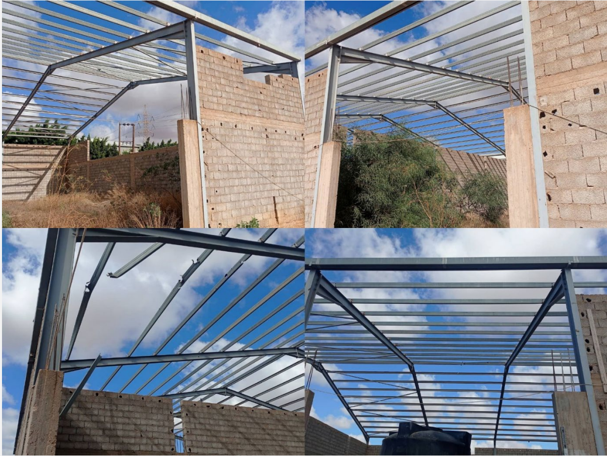
LRCS main warehouse in Benghazi (Bouatni area) prior to rehabilitation, showing structural damage and limited safety and operational capacity.
