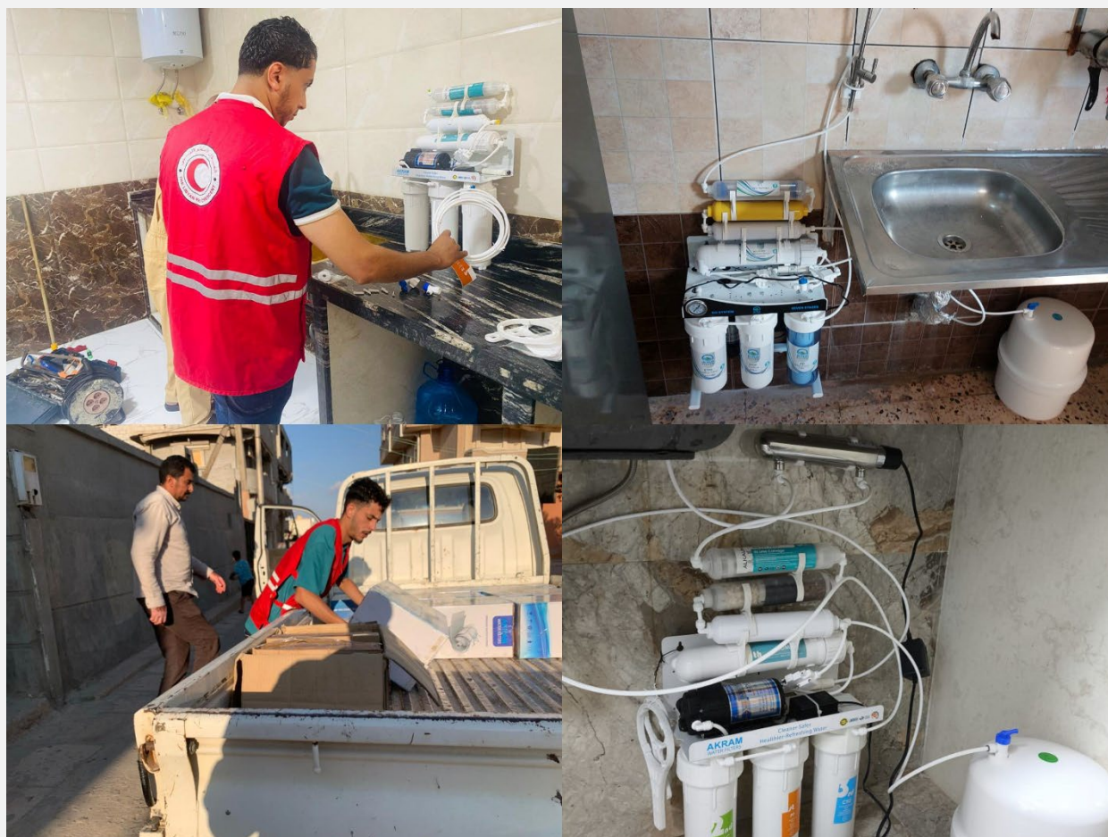
Trained LRCS volunteers assist in installing household Water purification Units in Shahat, Libya
