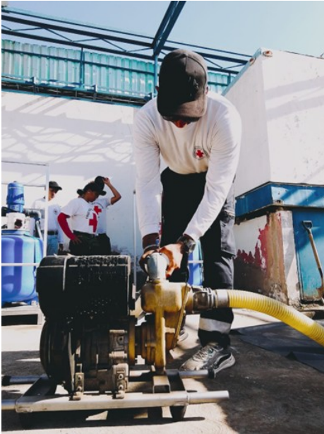
Start-up of a water treatment plant in the La Pedrera community. May 2026
