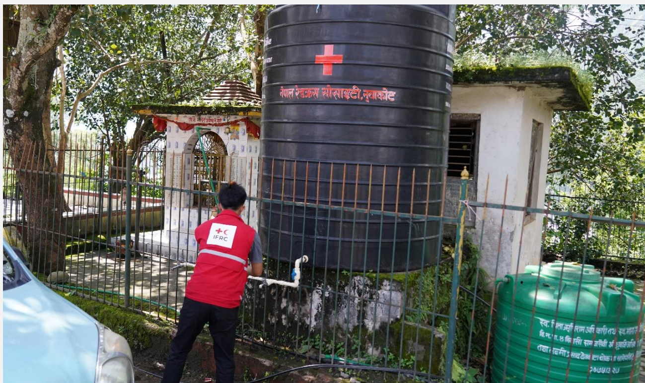
NRCS installing water storage tanks in different locations of Nuwakot to restore access to drinking water in the communities. (Photo: IFRC/Fleur)
