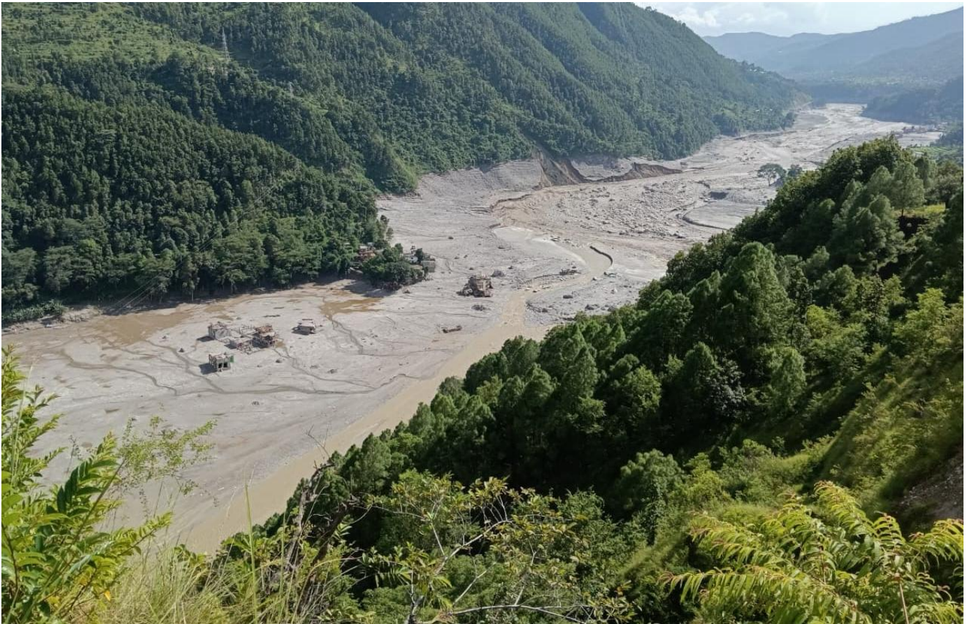
Houses, roads, and markets are swept away by the flash flood impacting Rasuwa, Nuwakot, and Dhading Districts. (Photo credit: Nepal Red Cross Society)
