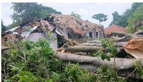
Fallen Cotton tree on houses caused by the minsstrom
