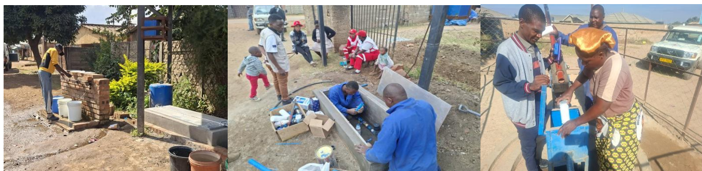
Figure 4: Installation of inline chlorinators in Budiro and Glen view, Harare, Zimbabwe, Photographer: Dorika Madzingiri, DFO*
