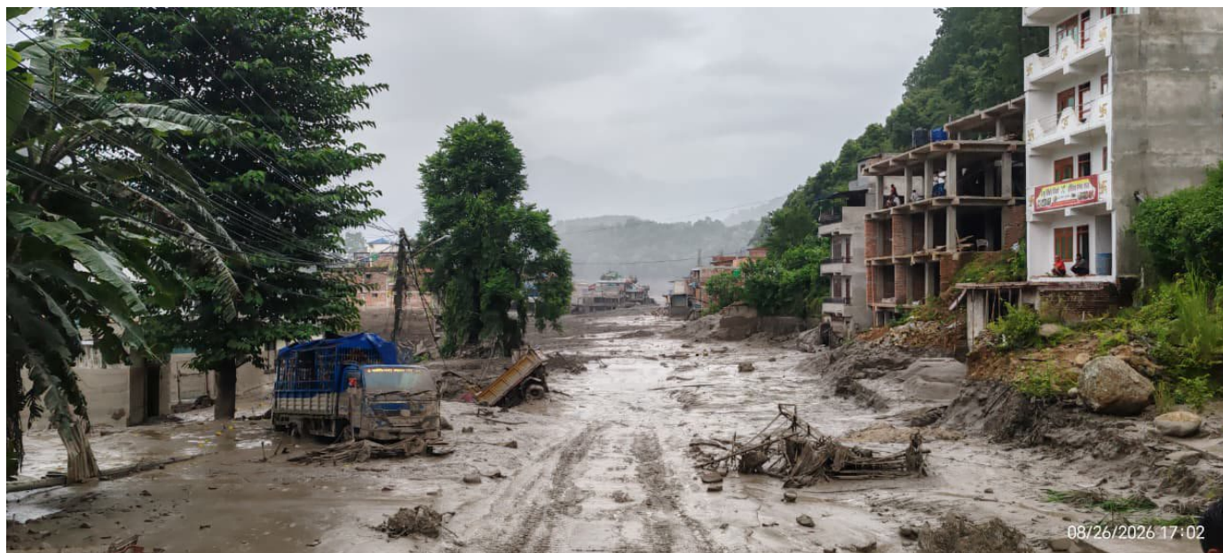
Roads, vehicles, and buildings damaged by the unprecedented flash flood in Nuwakot District. (Photo credit: Nepal Red Cross Society)
