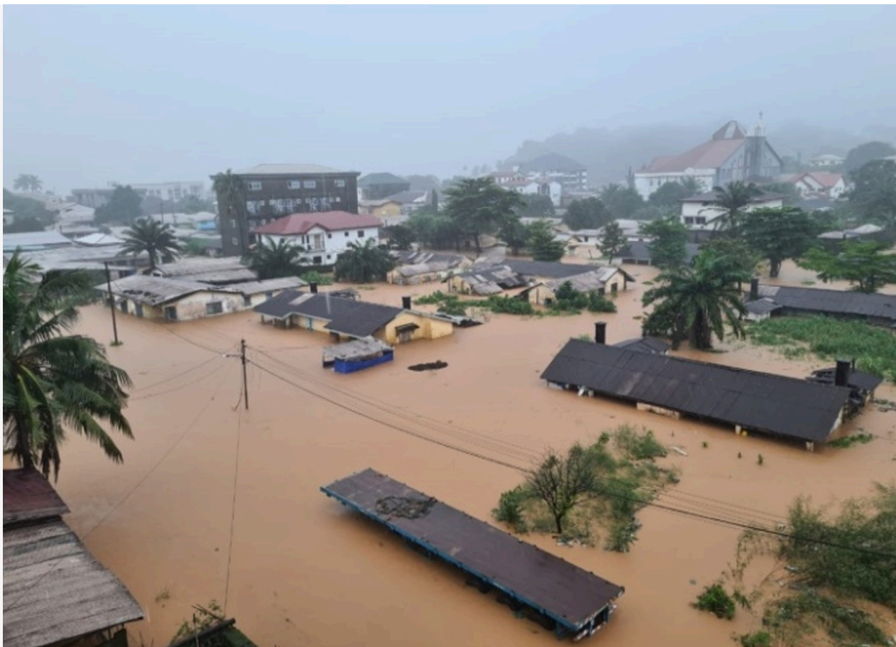
Houses completely affected by the flooding situation in Limbe
