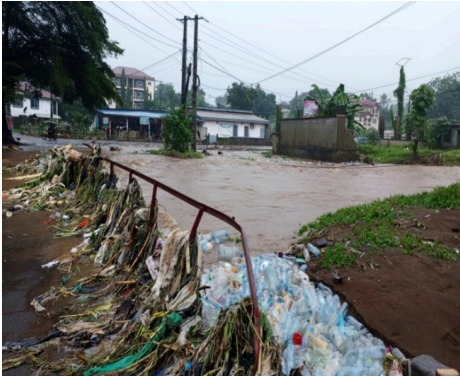
Jenguele channel overtopping its banks
