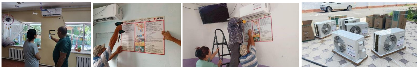
Picture 33, 34, 35 & 36 – Installation process of air conditioners, Jalal-Abad , Osh and Batken branches
