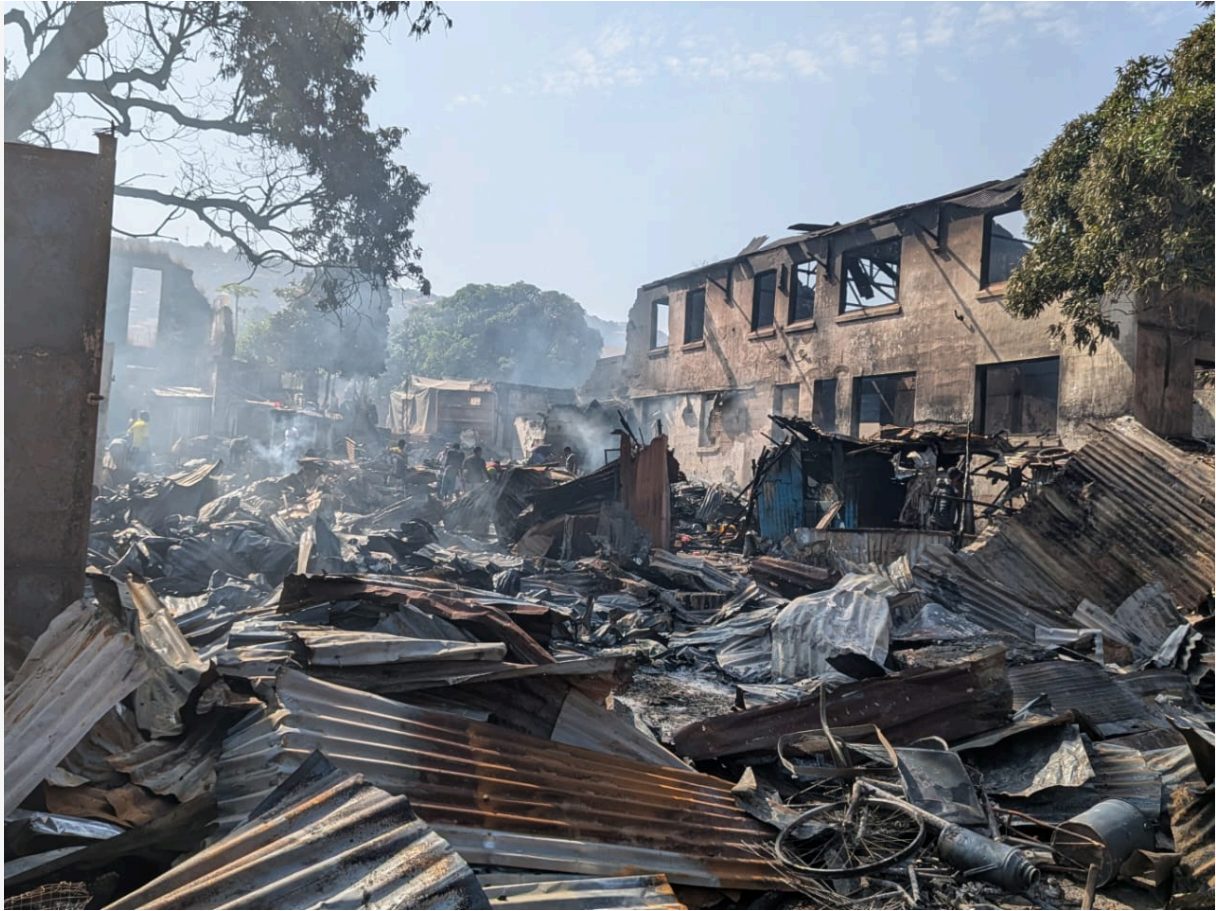
Fire impact in Freetown
