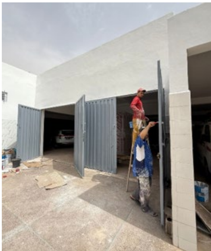
Photo12 -Rehabilitation works of Agadir Warehouse. Photo: MRCS
