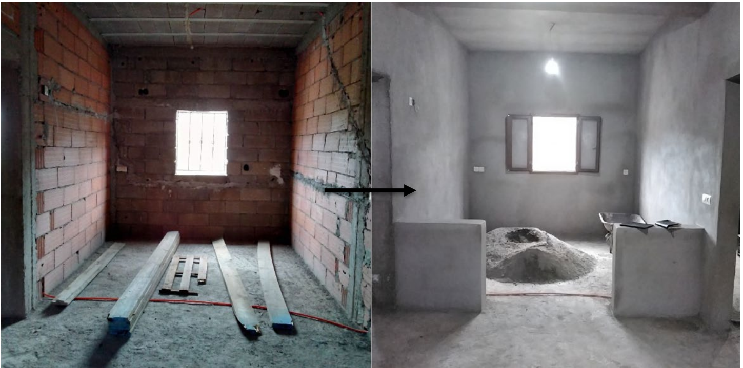
Photos 4 – Before and after photos of a house in Taroudant Province where a family completed finishing works using top-up cash assistance under the Rapid Cash for Shelter Programme by MRCS/IFRC, complementing government reconstruction support. Photos: MRCS
