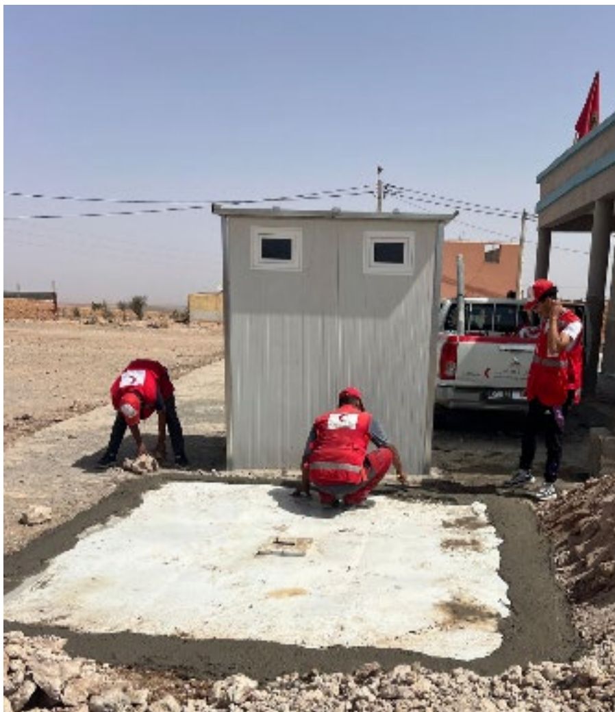
Photo 9 - Installation of toilets modules in El Haouz (September 2025). Source MRCS
